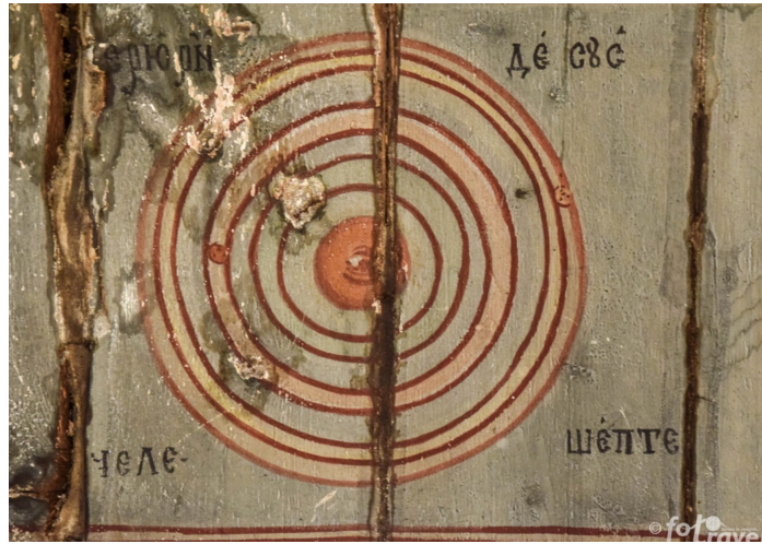
Fig. 3: The ceiling of the Uniate church in Șurdești (Maramureș County, photo 2016)
