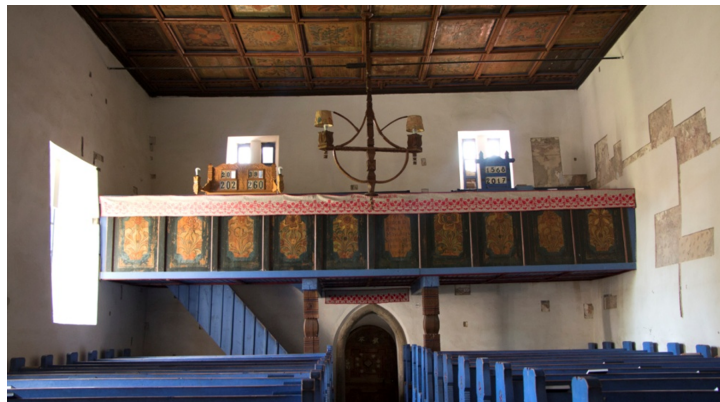
Fig. 4: The interior of the Unitarian church in Ocland (Harghita County), with a coffered ceiling.
