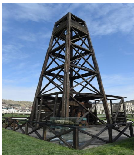
Fig. 2. A replica of the world's first drilled oil well derrick; drilled at Bibi-Heybat, Baku, in 1846 [Azernews, N31 (1233) April 28 – 2 May 2017, p.1].
